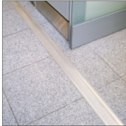
Interior Joints Boxes / Suites
