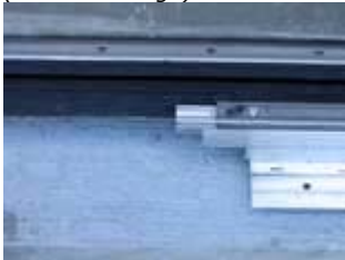
Sliding components of the MIGUTAN mounting legs are staggered and slipped over adjoining sections to ensure positive alignment.
